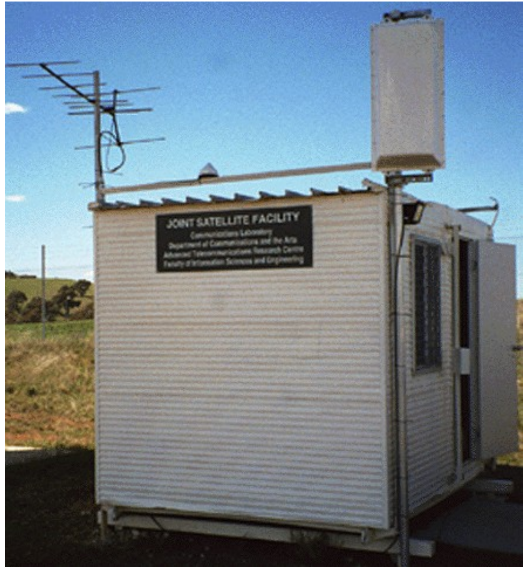
Picture 20 - Translator Site with antennas (L-R VHF Ch 8-H, GPS, UHF Ch 44-V)
